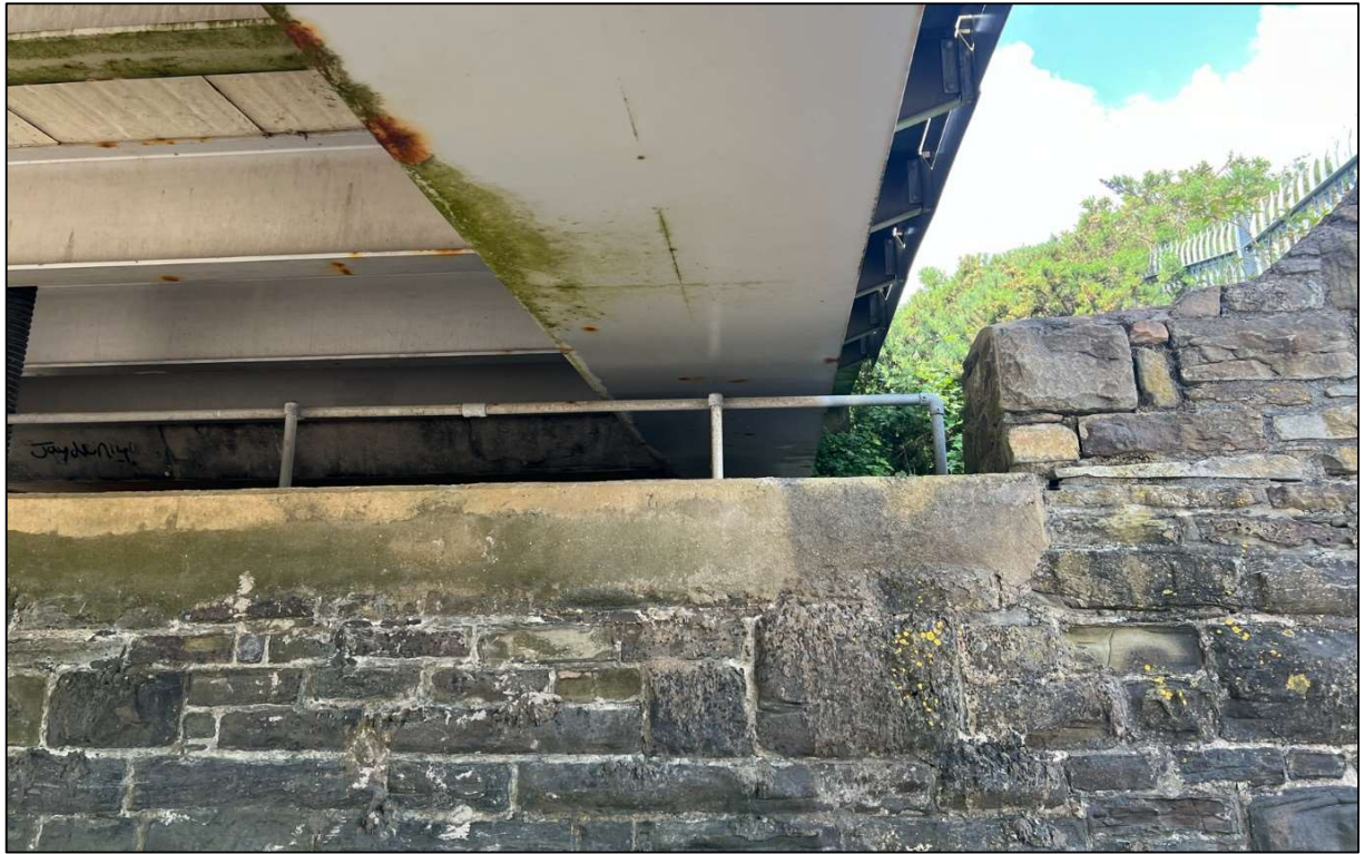
Figure 7: Upper section of the western abutment.
