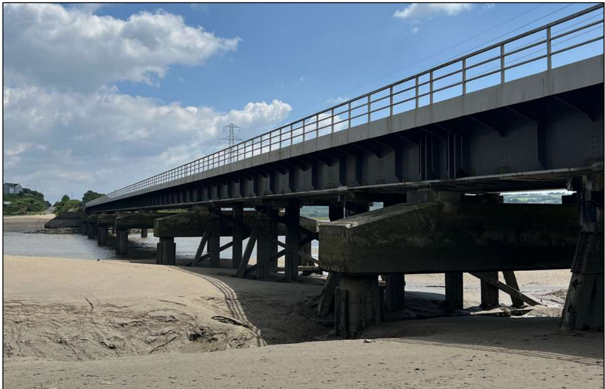
Figure 6: View of rail crossing during low tide.
