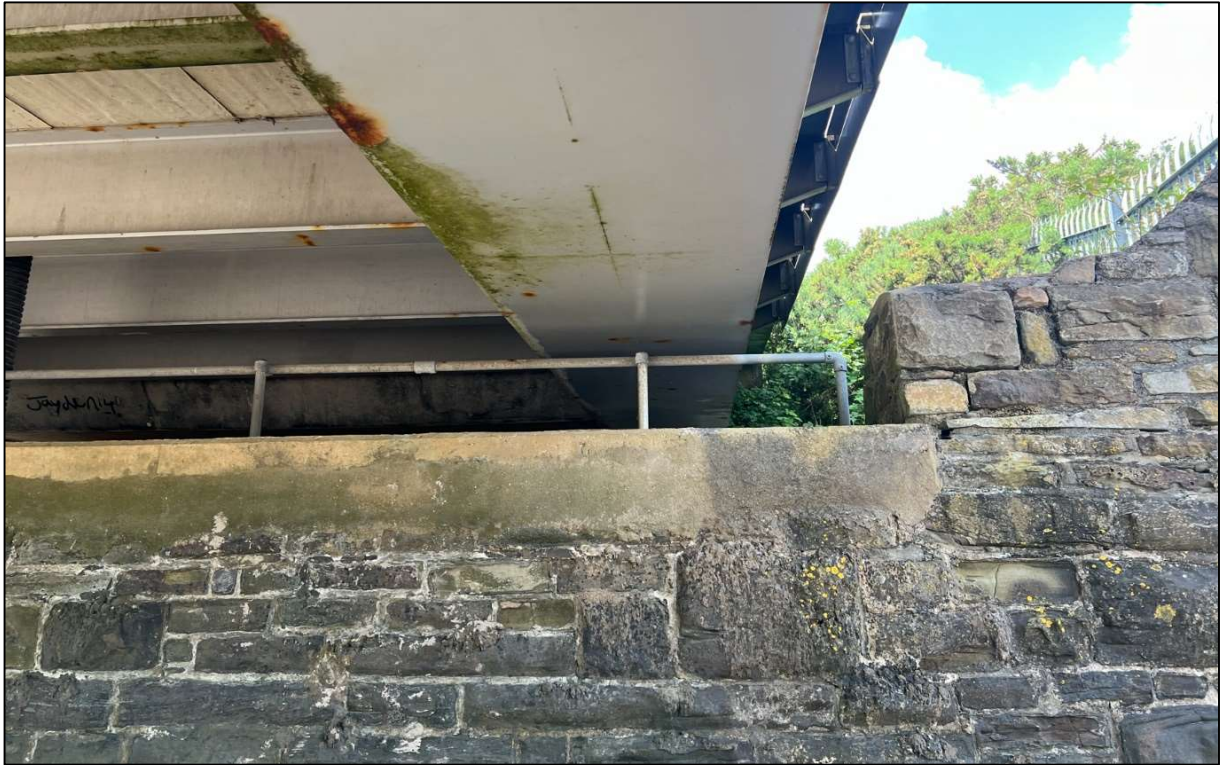
Figure 6: Upper section of the western abutment.
