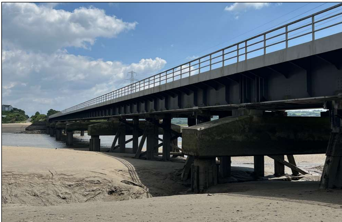
Figure 5: View of rail crossing during low tide.
