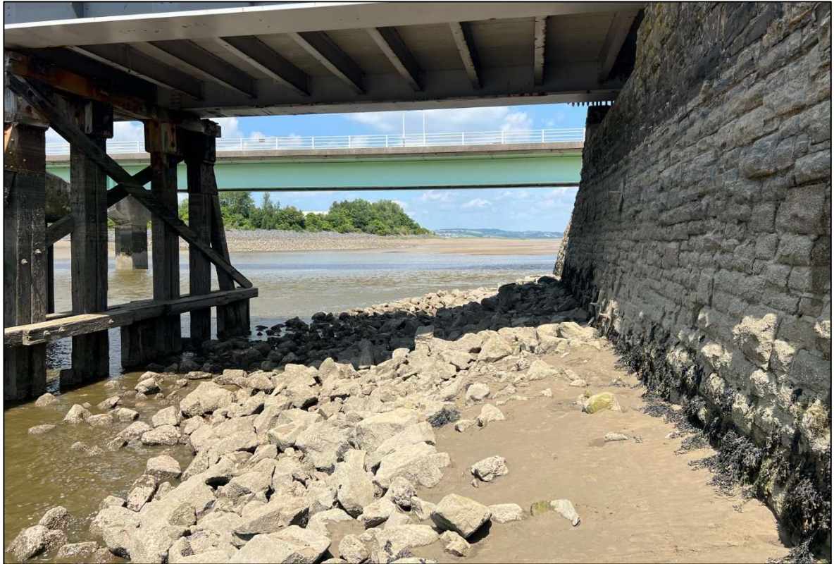
Figure 8: Eastern abutment during low tide.
