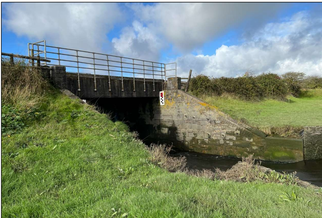
Figure 2: Abutment of Section A (west shore).
