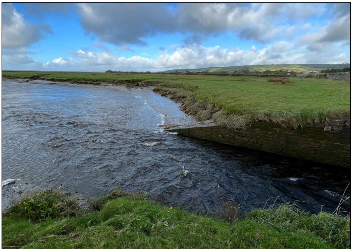
Figure 7: Downstream side of the structure flowing into the wider estuary.
