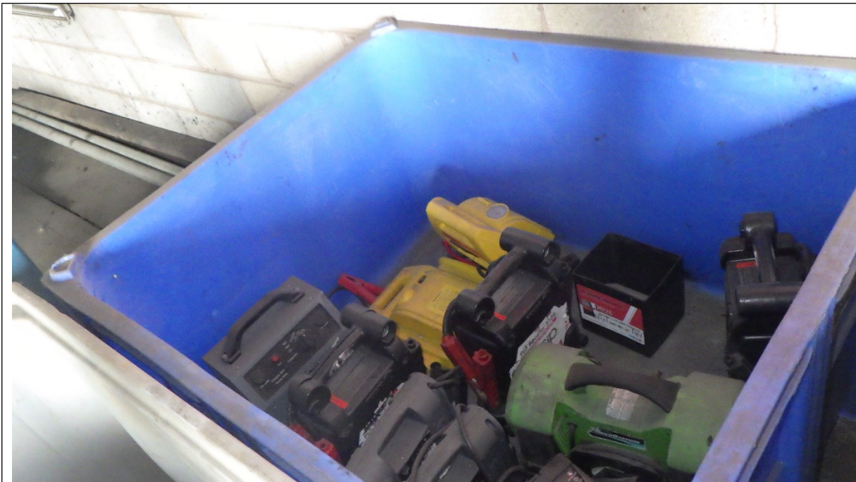
Enclosed battery storage.
