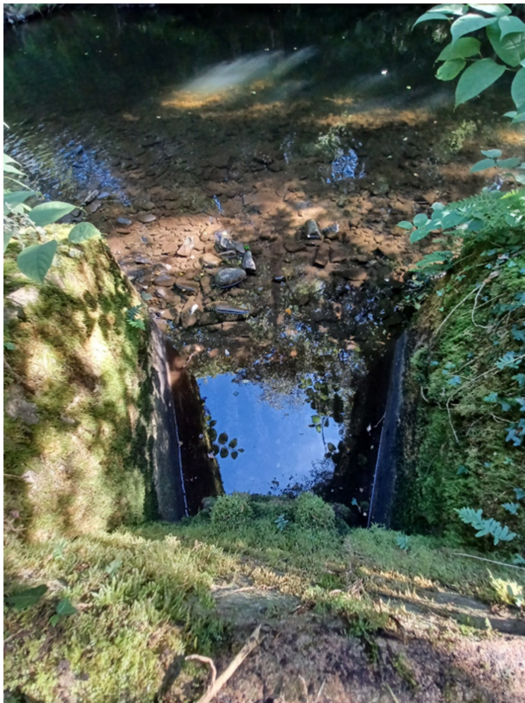
Figure 8 – storm discharge point (A2 & A3)
