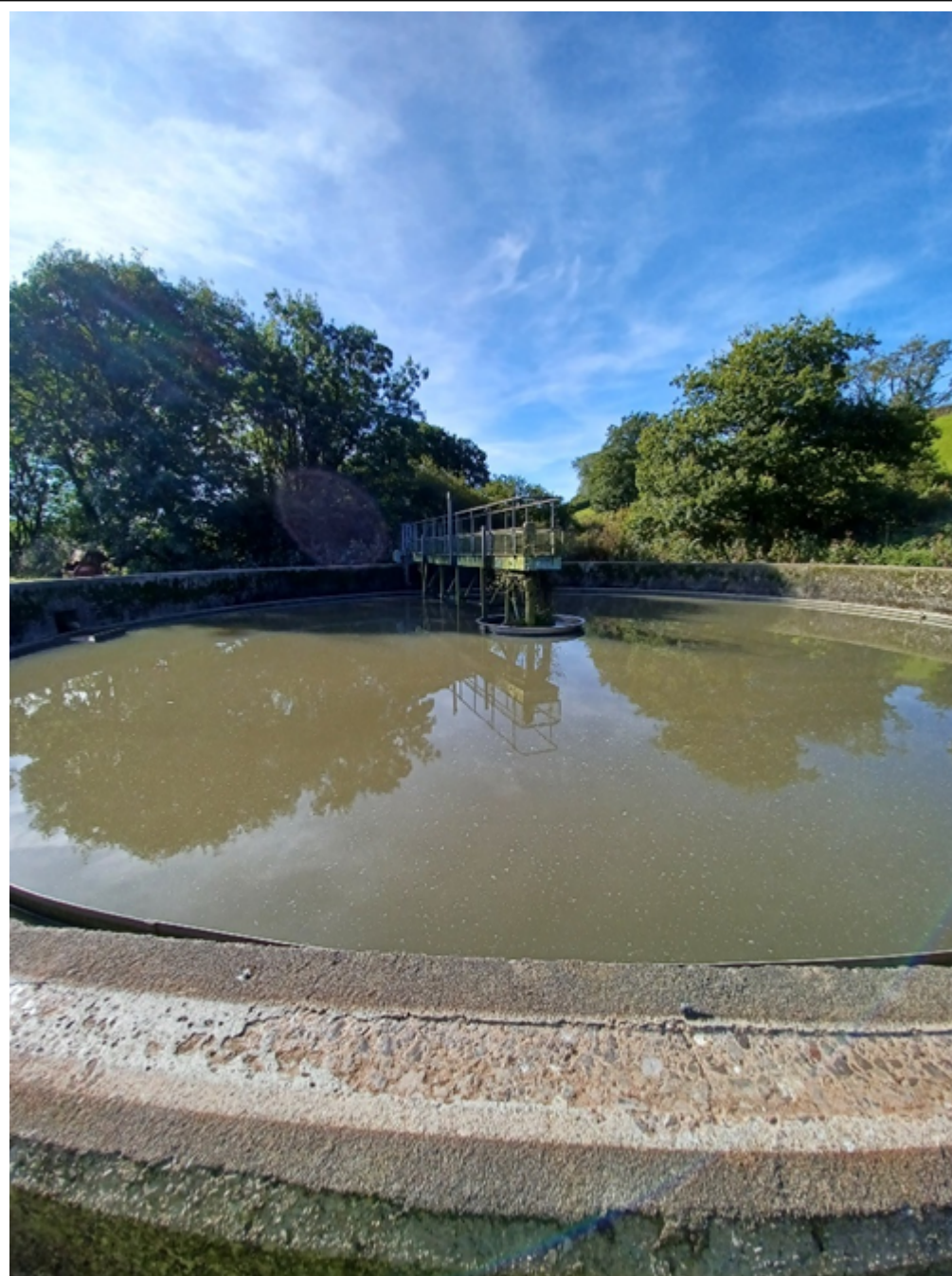
Figure 2 – Primary settlement tank
