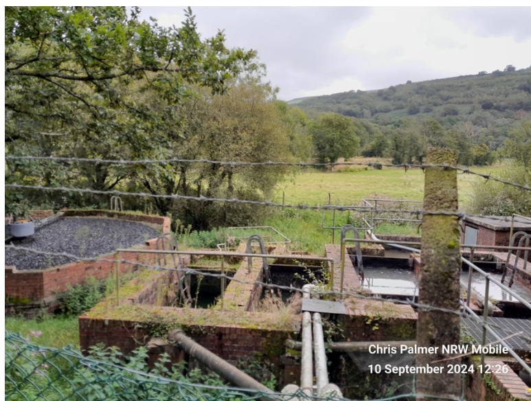
Two primary settlement tanks (on the left)
