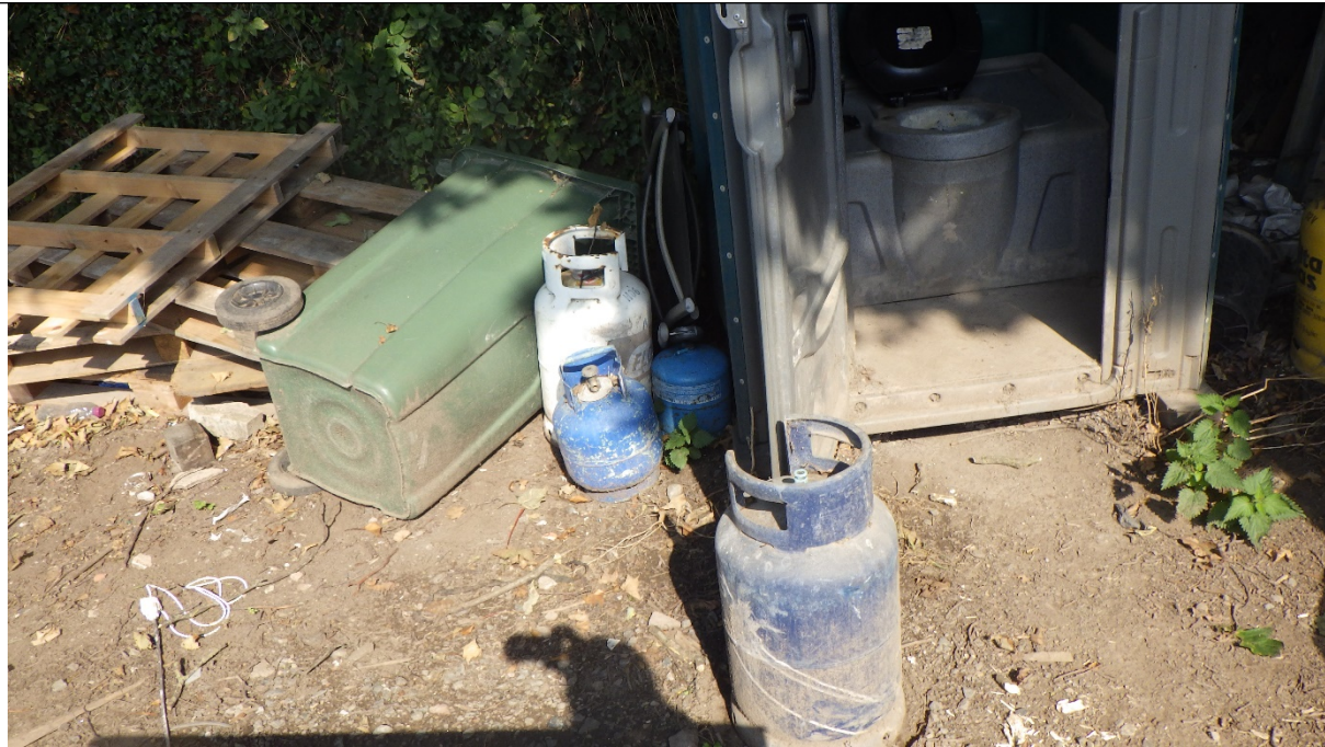
Gas bottles stored outside and not secure.
