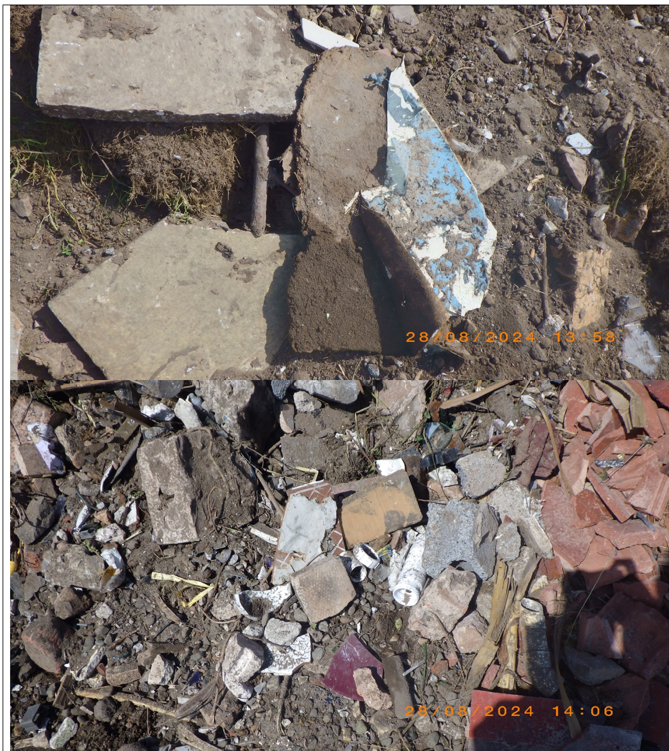
Photographs showing waste deposited on site
