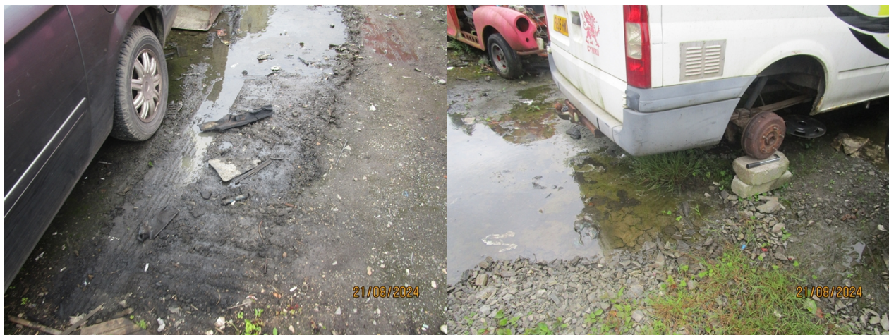
Figure 4. hardstanding rutted and with standing water
