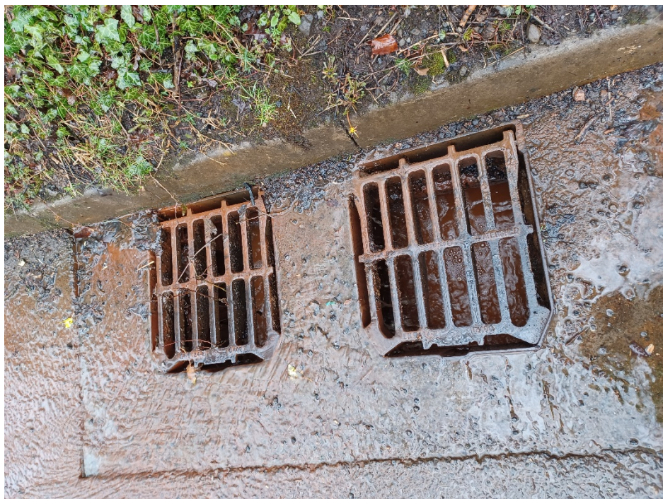
Figure 4: discoloured water entering highway drain.
