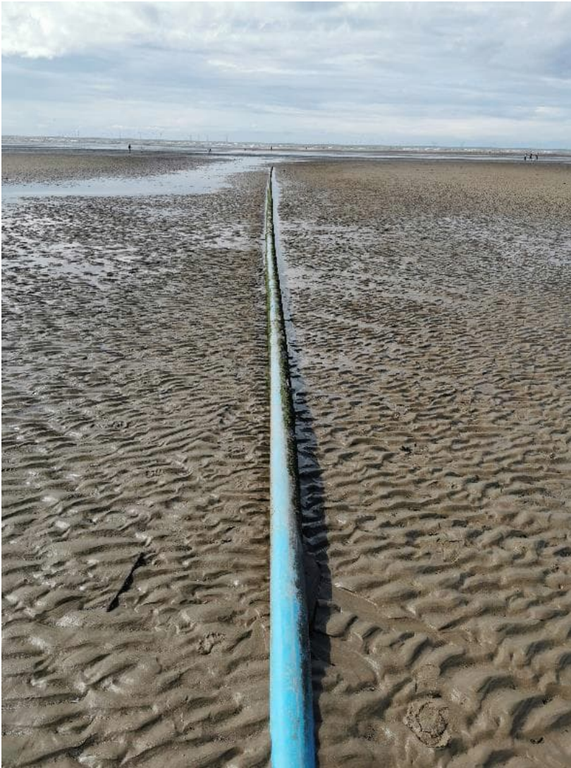
Figure 1.2: Pipeline running across beach surface
