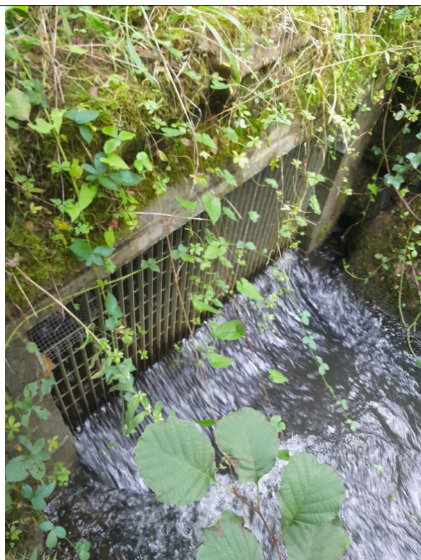
Photograph 1: Outfall from the Turbine House
