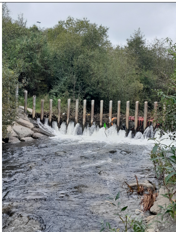
Photograph 3: Groynes with Debris
