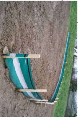
TYPICAL SILT FENCE CONSTRUCTION
