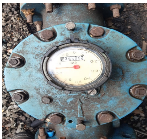
Figure 2: Turbine meter
