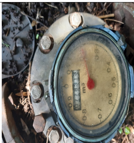
Figure 2: Turbine meter
