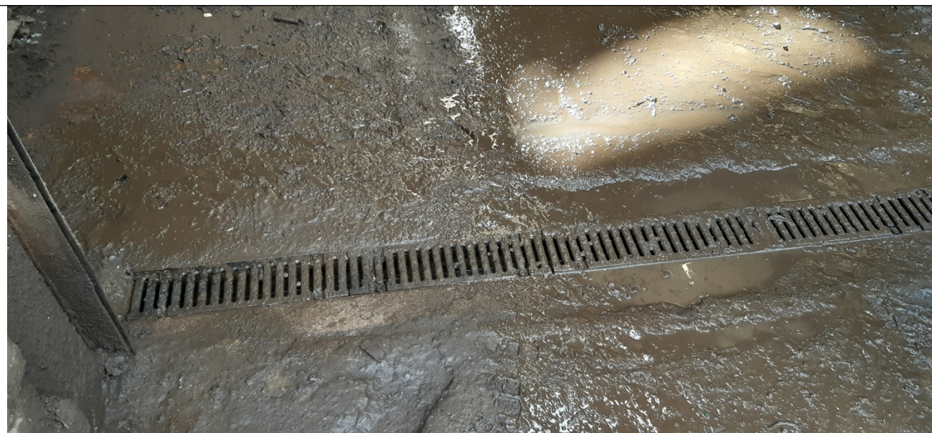
Photo 8 - Drainage channels at Green Steel Ltd
