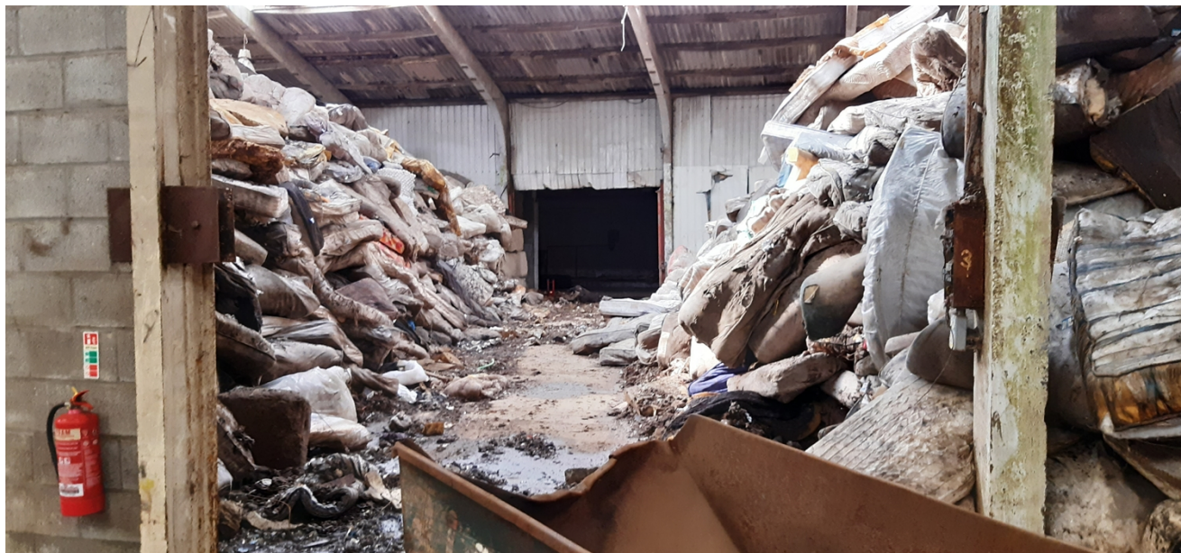
Photo 10 - Unprocessed mattresses with fire break at Green Steel Ltd
