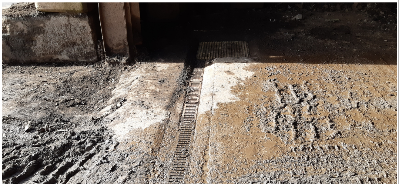
Photo 7 - Drainage channels at Green Steel Ltd
