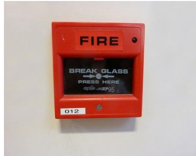
Figure 2.0 - Manually Operated Fire Call Point
