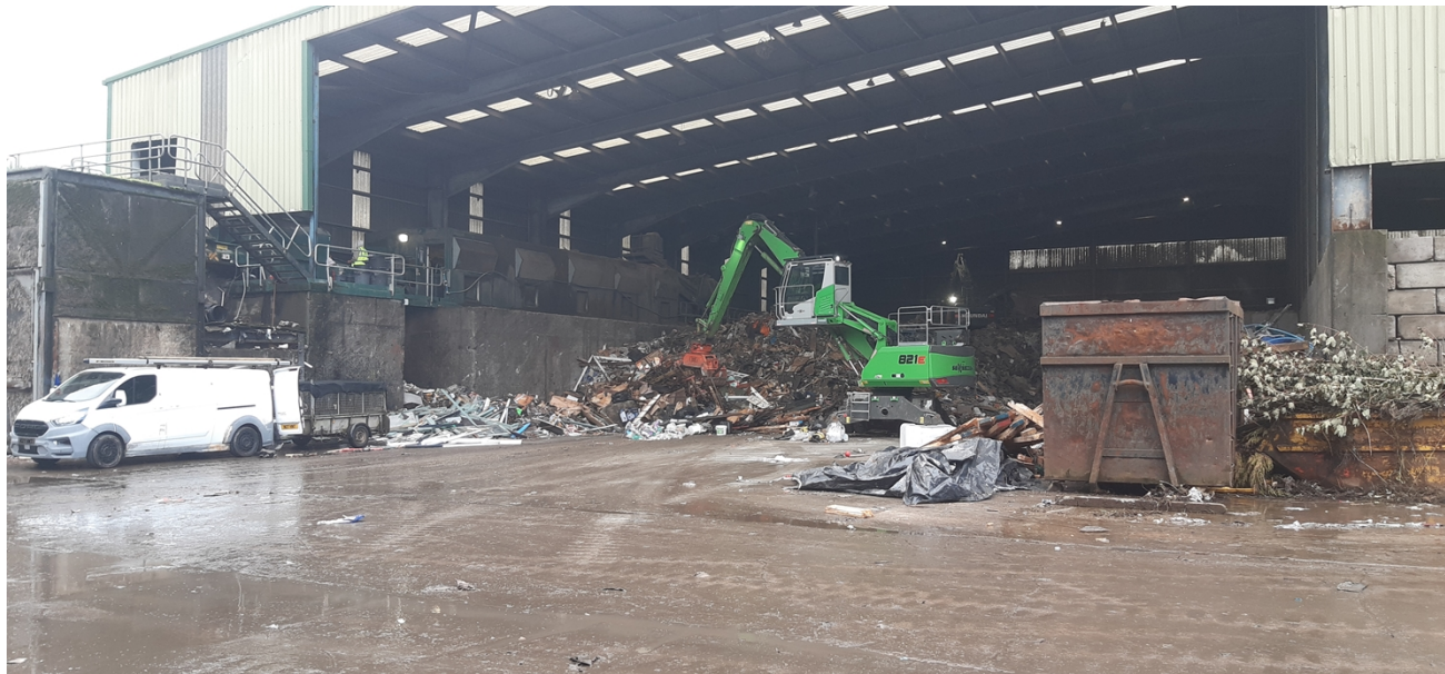
Photo 1 - View inside waste transfer station building
