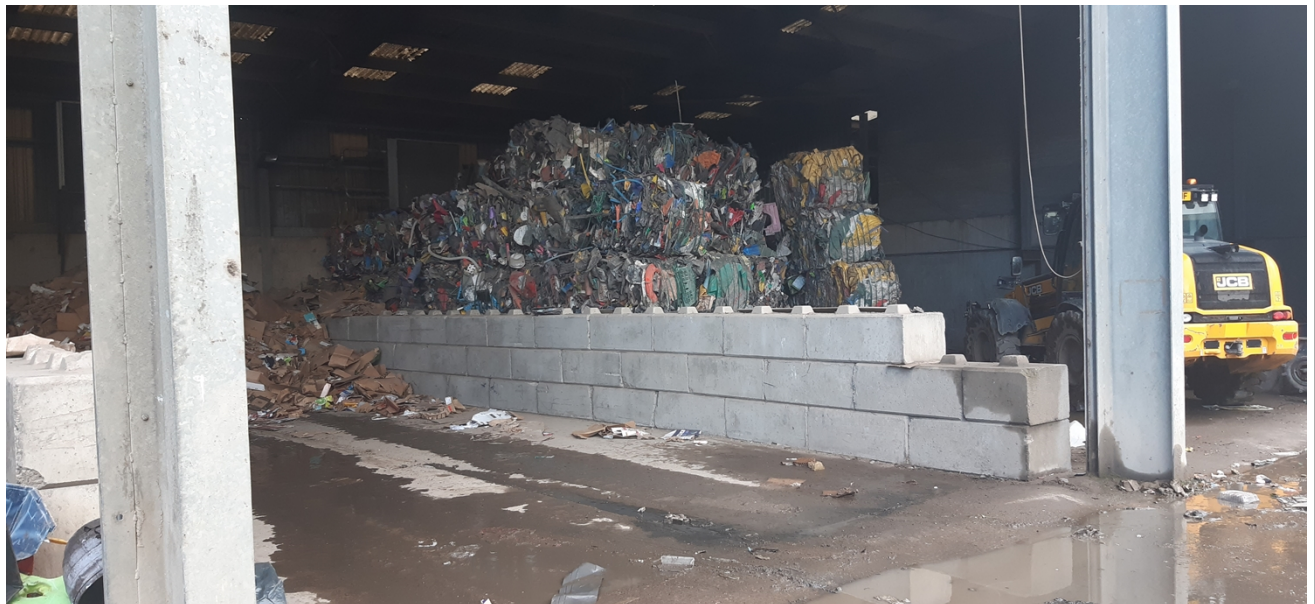
Photo 3 - View inside waste transfer station building drying sheds
