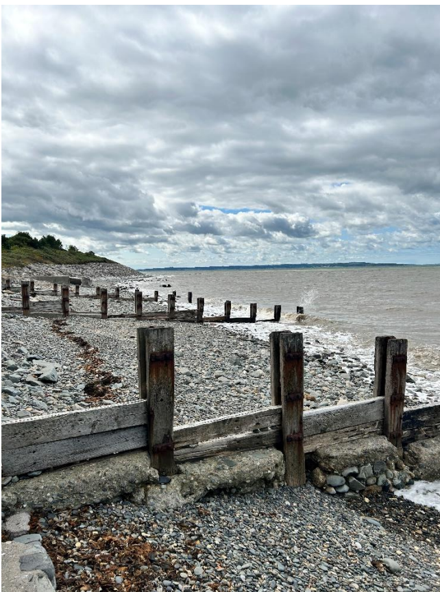
Photo 4 – wooden and metal sleeper groins on pebble beach looking west towards grassy headland.
