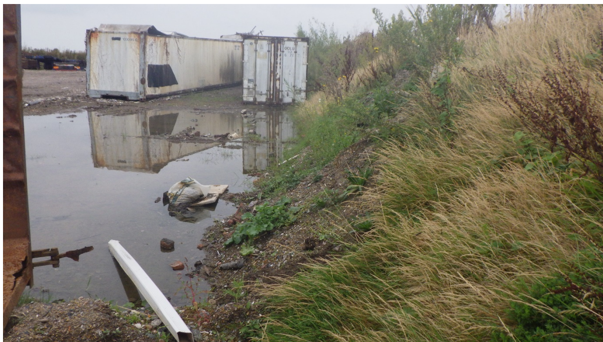
Bund created with trommel fines on site
