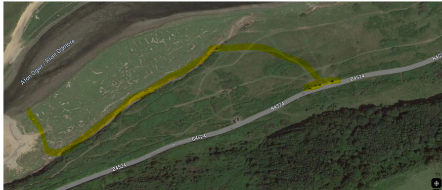
Figure 2 Showing track area for excavators to the river
