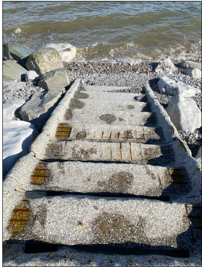
PHOTO 1 - OVERALL VIEW OF BOTTOM STAIRCASE
