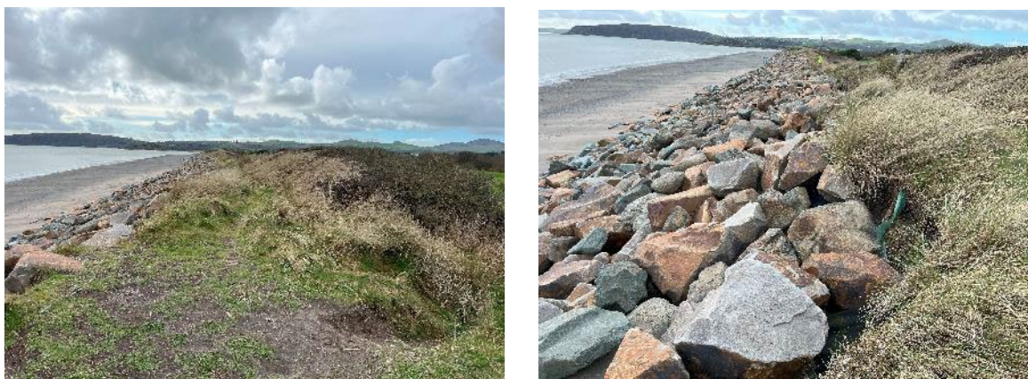
Figure F10. Area with high vegetation. Left: Looking towards the West. Right: Looking towards the West.
