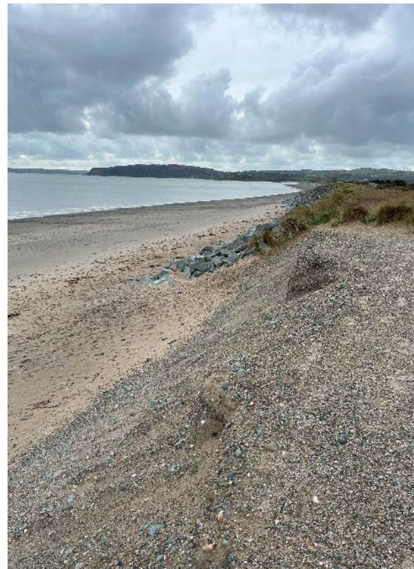
Figure F3. Renourishment area to the East of the Eastern end of the revetment. Left: Looking East Right: Looking West
