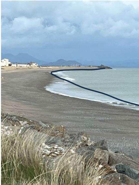
Figure F14. Looking towards the East half way from the revetment
