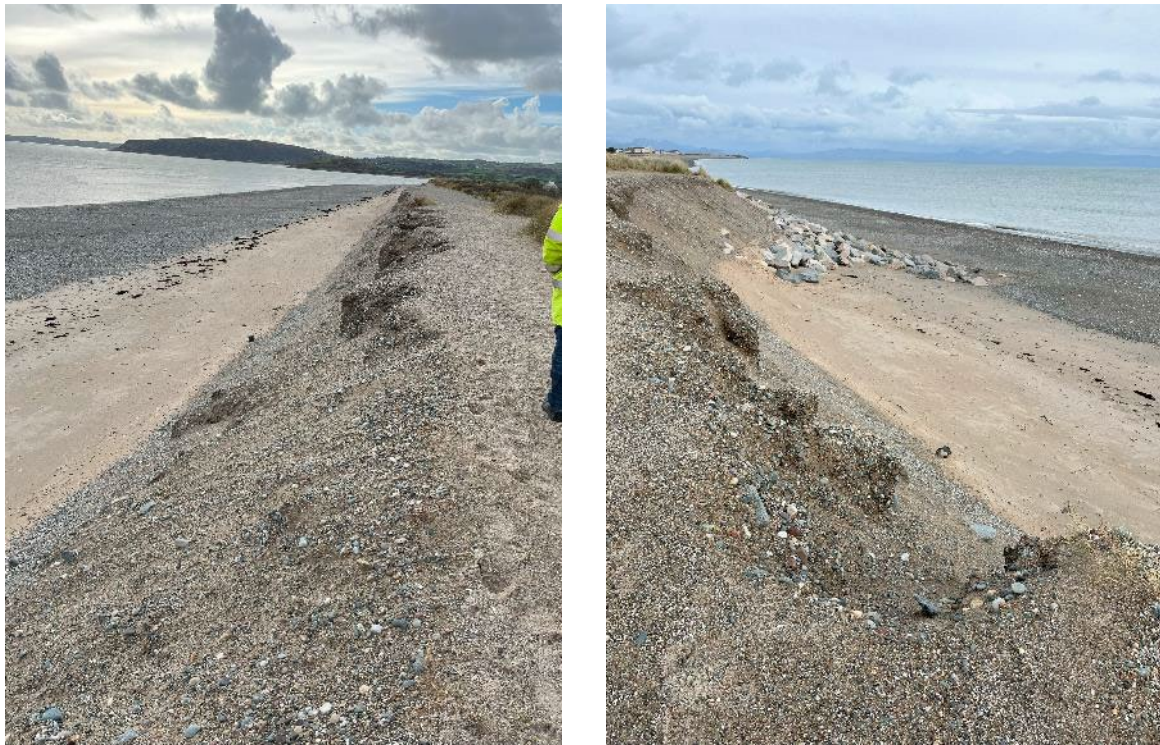
Figure F13. Renourishment in the Westen area (to the West of the revetment) Left: Looking towards the West. Right: Looking towards the East.
