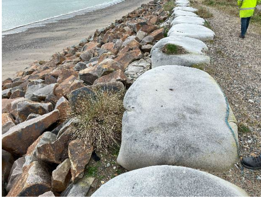
Figure F6. Repair work with bags full of dredged sediment
