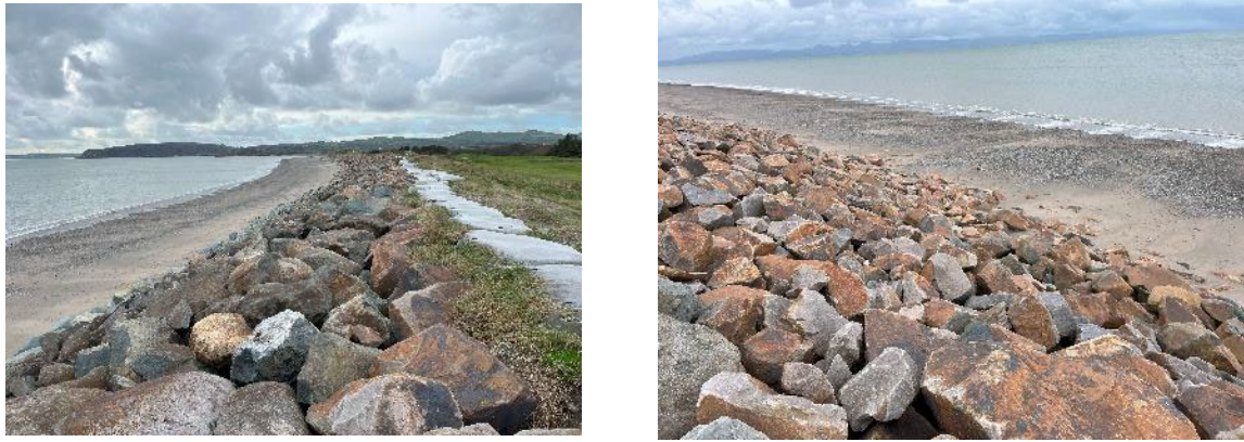
Figure F8. Left: Looking West. Right: looking down on to the beach towards the East
