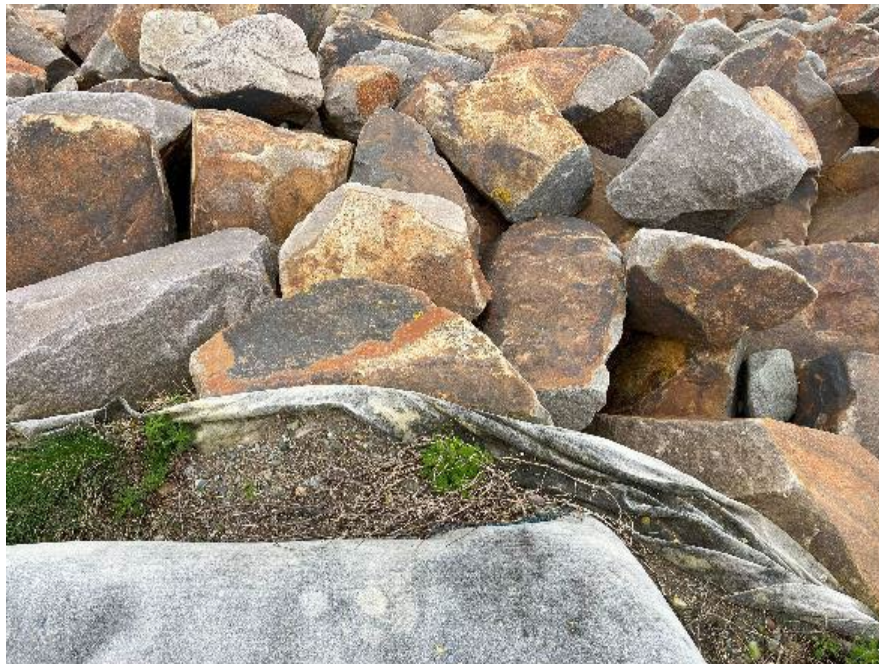
Figure F7. Geotechnical material coming through the rocks
