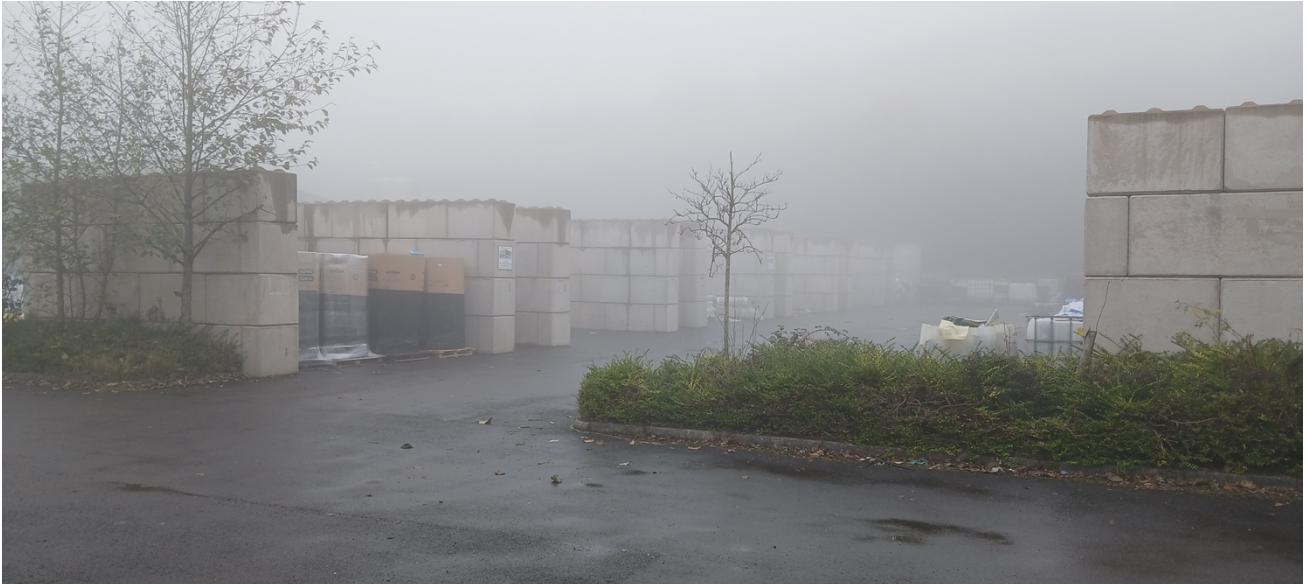
Photo 1 - Plastic waste(s) stored in compliance with the sites FPMP document
