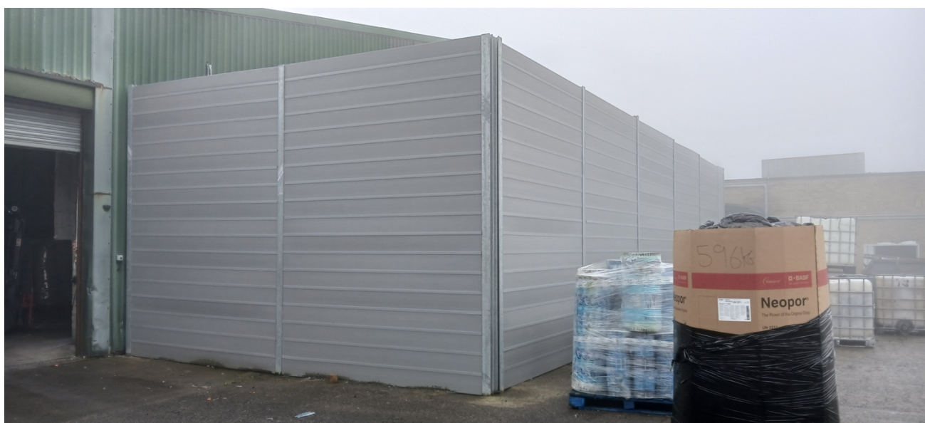
Photo 4 - Recently installed noise barrier to mitigate excess noise
