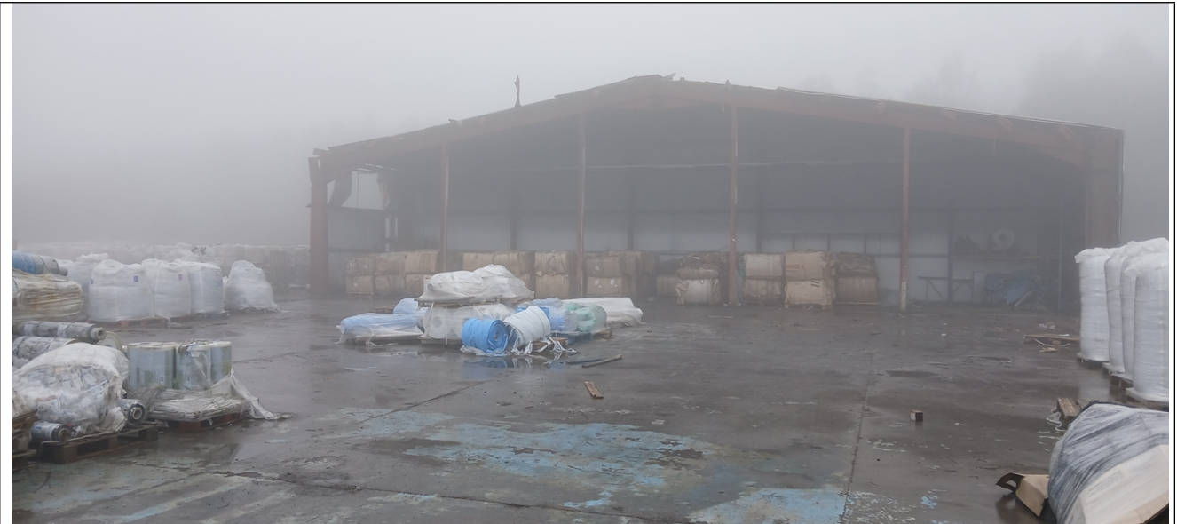
Photo 5 - Waste(s) stored to rear of the building
