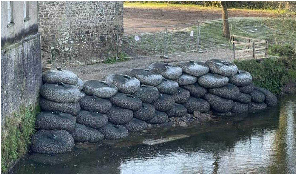
Figure 3-2: Emergency repair works to wall failure
