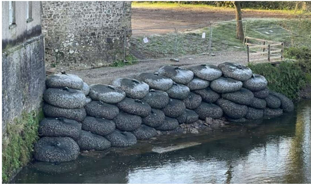
Figure 1 – Emergency stabilisation works using 48 no. Salix Aqua Rock Bags carried out 28/11/23 – 29/11/23.
