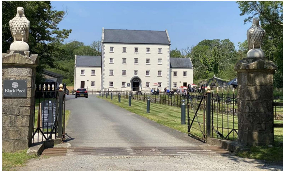
Figure 3 – Southern entrance to Black Pool Mill to be used by construction traffic.
