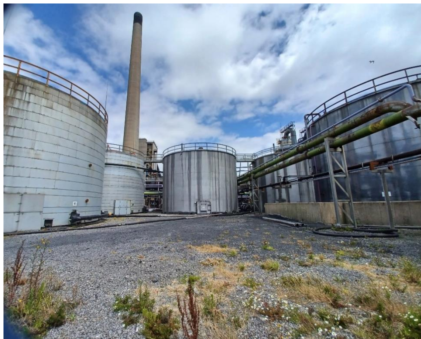
Image 3: Tank Farm - Coal Tar (left), Ammonia Liquor (rear) and Effluent (right)
