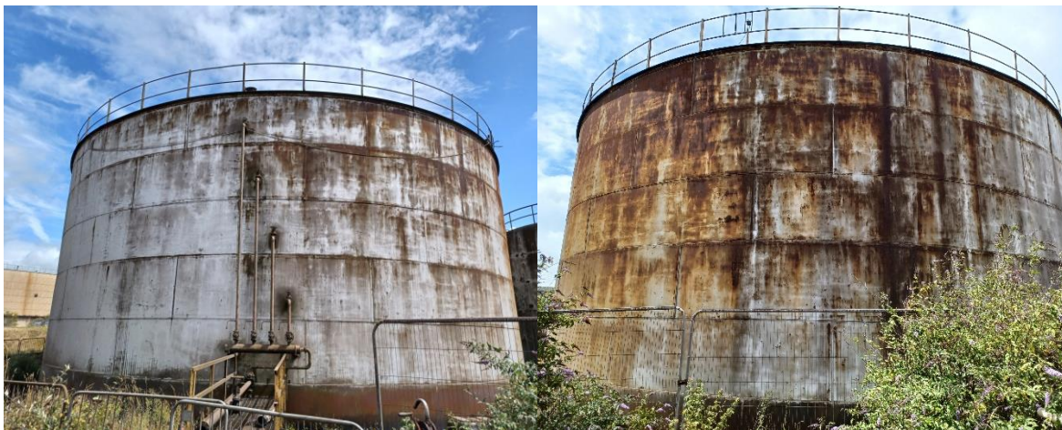
Image 5: Million Gallon Tank (MGT) - North (left) and South (right)
