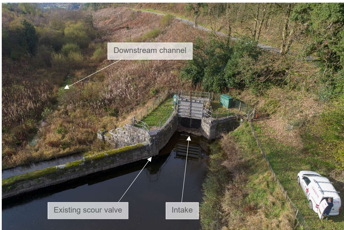
Figure 2-1 – Intake on the River Marchnant (Source: North Midlands Construction 31/10/18)
