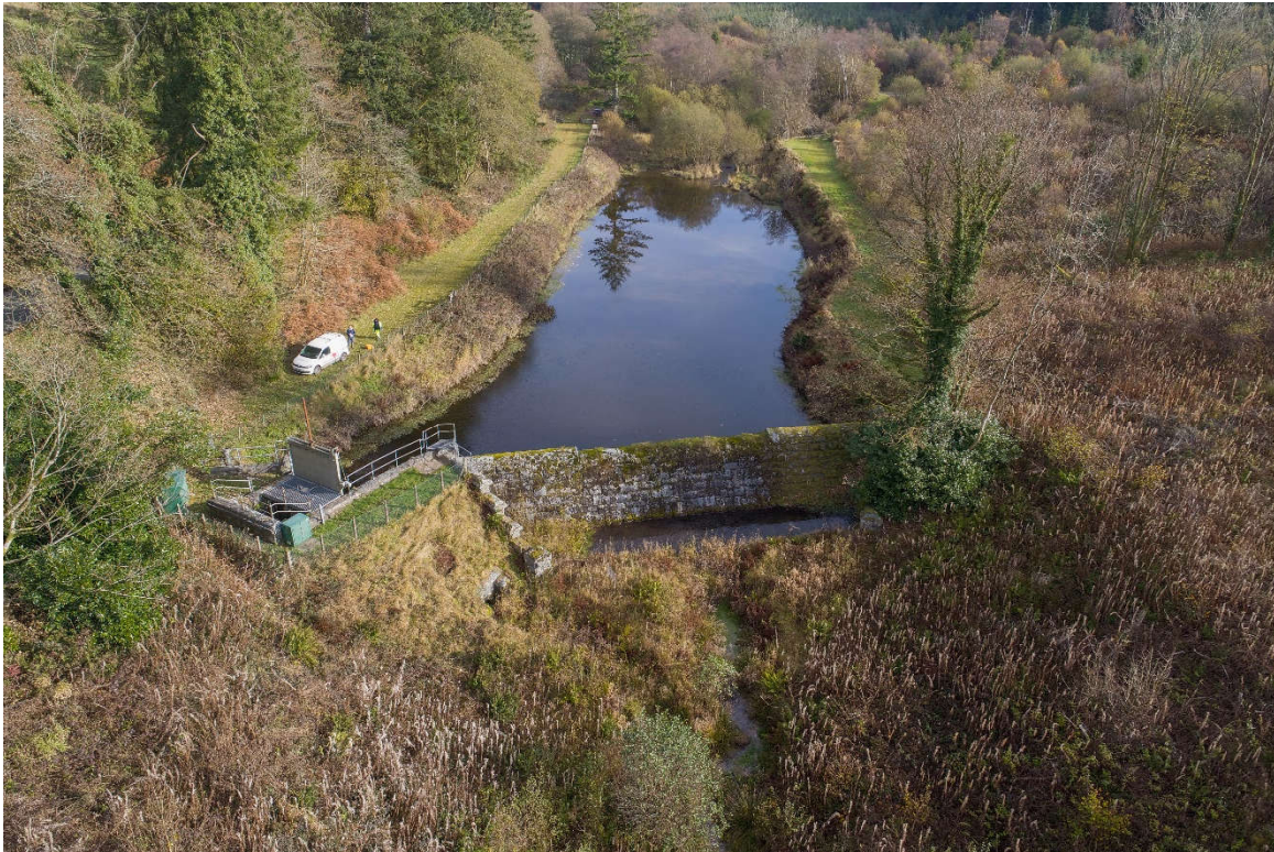
DJI_0252-HDR – Drone image taken looking upstream showing the stagnant channel immediately downstream, the weir structure and the weir pool (MAR002 and MAR003) (Source: North Midlands Construction 31/10/18).
