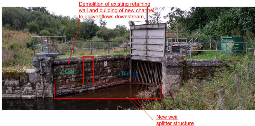
Figure 4-2 – Photographic illustration of Marchnant intake structure
