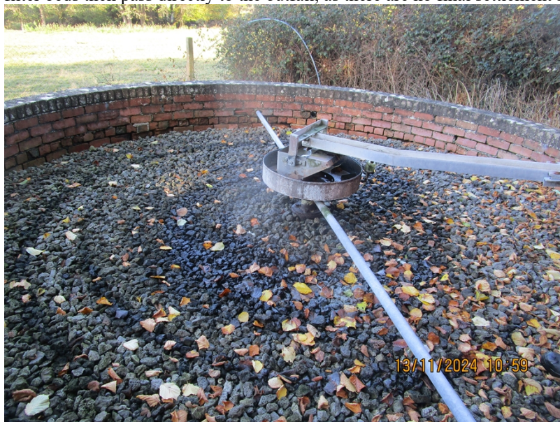
Outfall and sampling point
