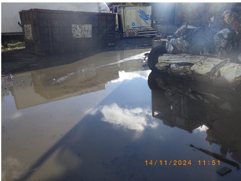
image of pooling water on site due to blocked drain.
