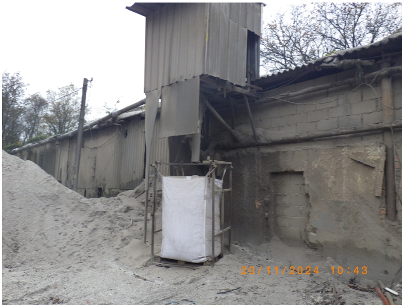
image of dust collection system at rear of site.
