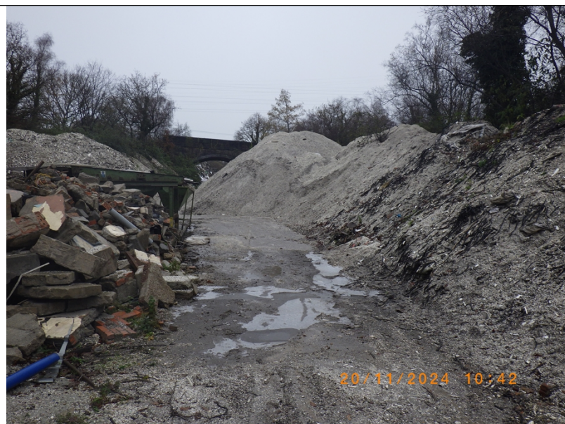
Image of waste storage at the rear of the site.
