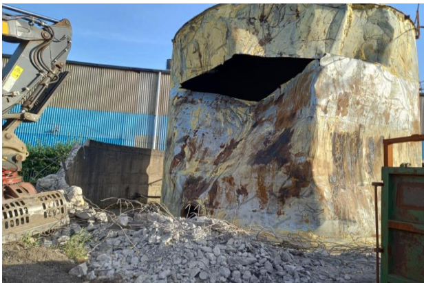
Photograph C-10: Removal of AST
