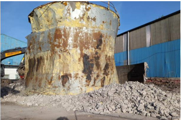
Photograph C-7: Secondary containment removed
