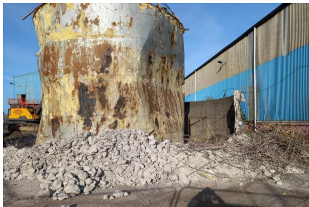
Photograph C-9: Removal of AST
