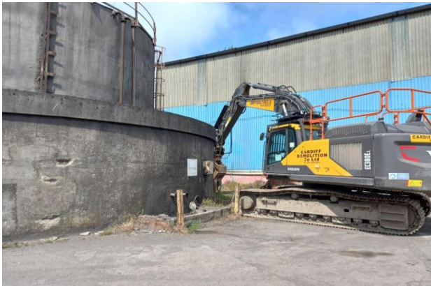
Photograph C-6: Removal of secondary containment
