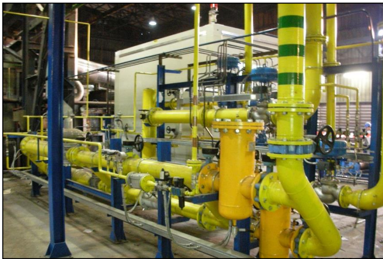
Preassembled gas train (analogy)
