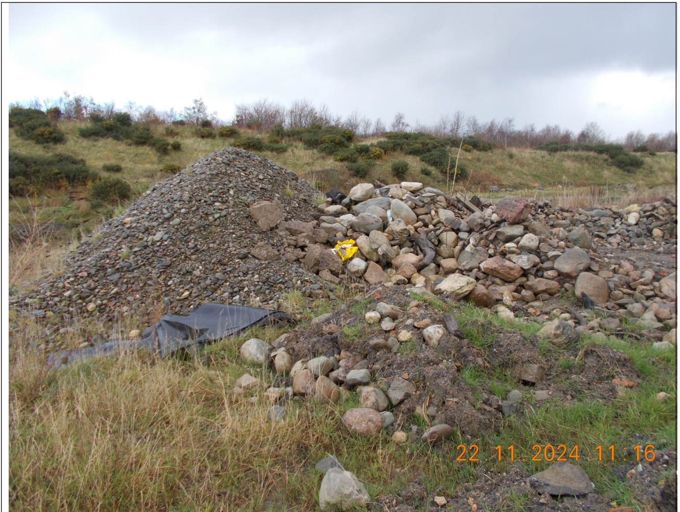
Photographs showing waste storage on site
