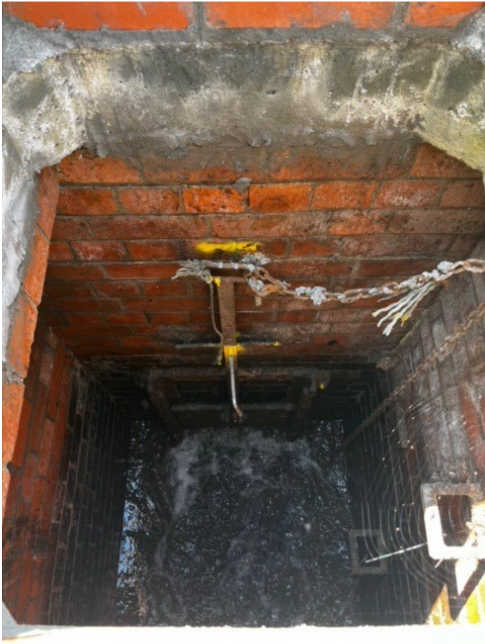
Image 2: Penstock downstream of inlet
