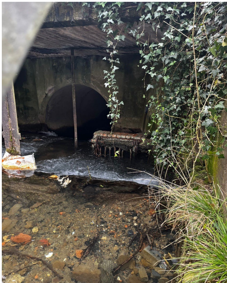
Image 1: 1.8M Culvert adjacent to 450mm inlet with brick headwall
