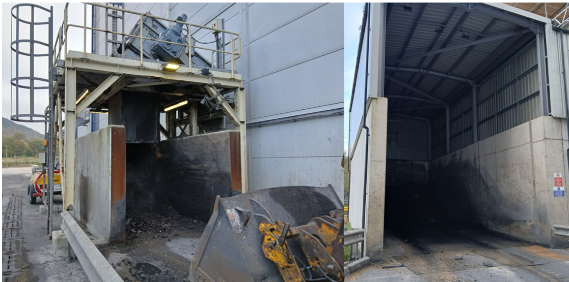
Left: IBA chute from inside plant Right: IBA bulk storage area
