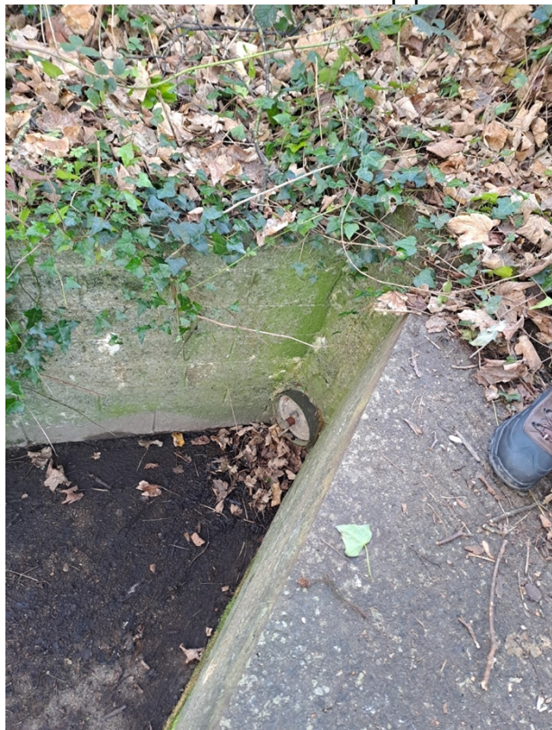
Image 4 - Bung at the outfall
