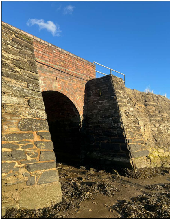
Figure 4: Estuary side of underbridge.
