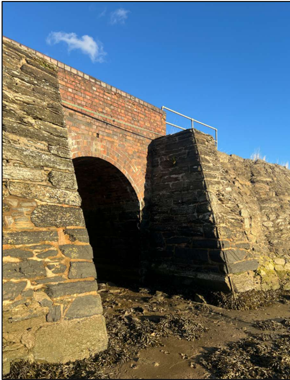
Figure 10: Estuary side of underbridge.
