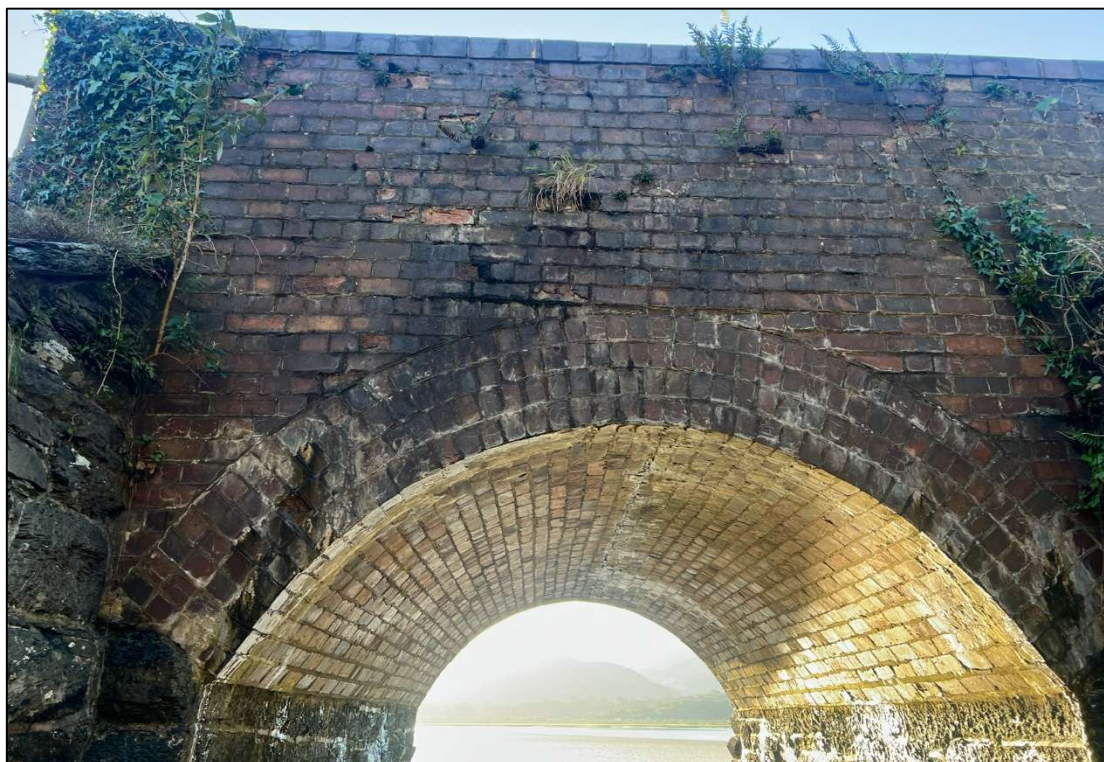
Figure 1: View of masonry underbridge arch.
