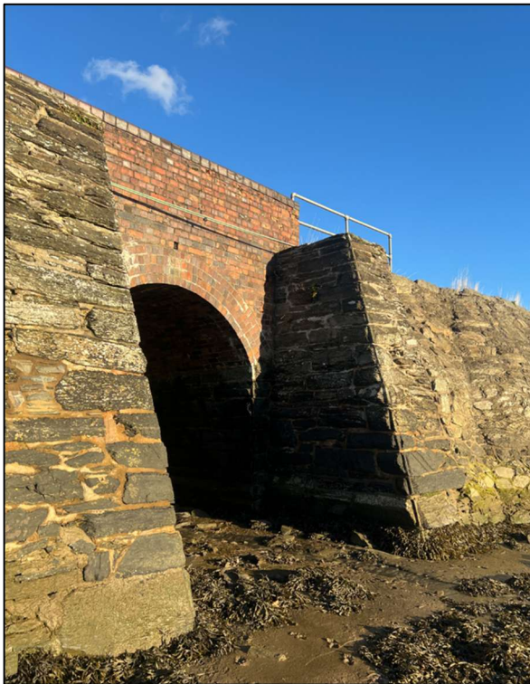
Figure 6: Estuary side of underbridge.
