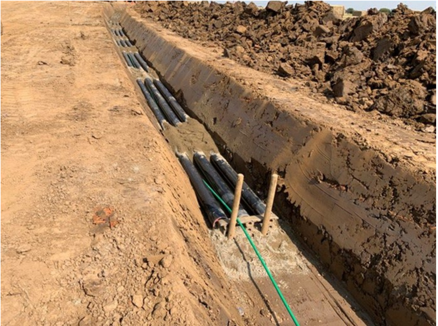
Figure 3.18: Example of an onshore export cable trench.
