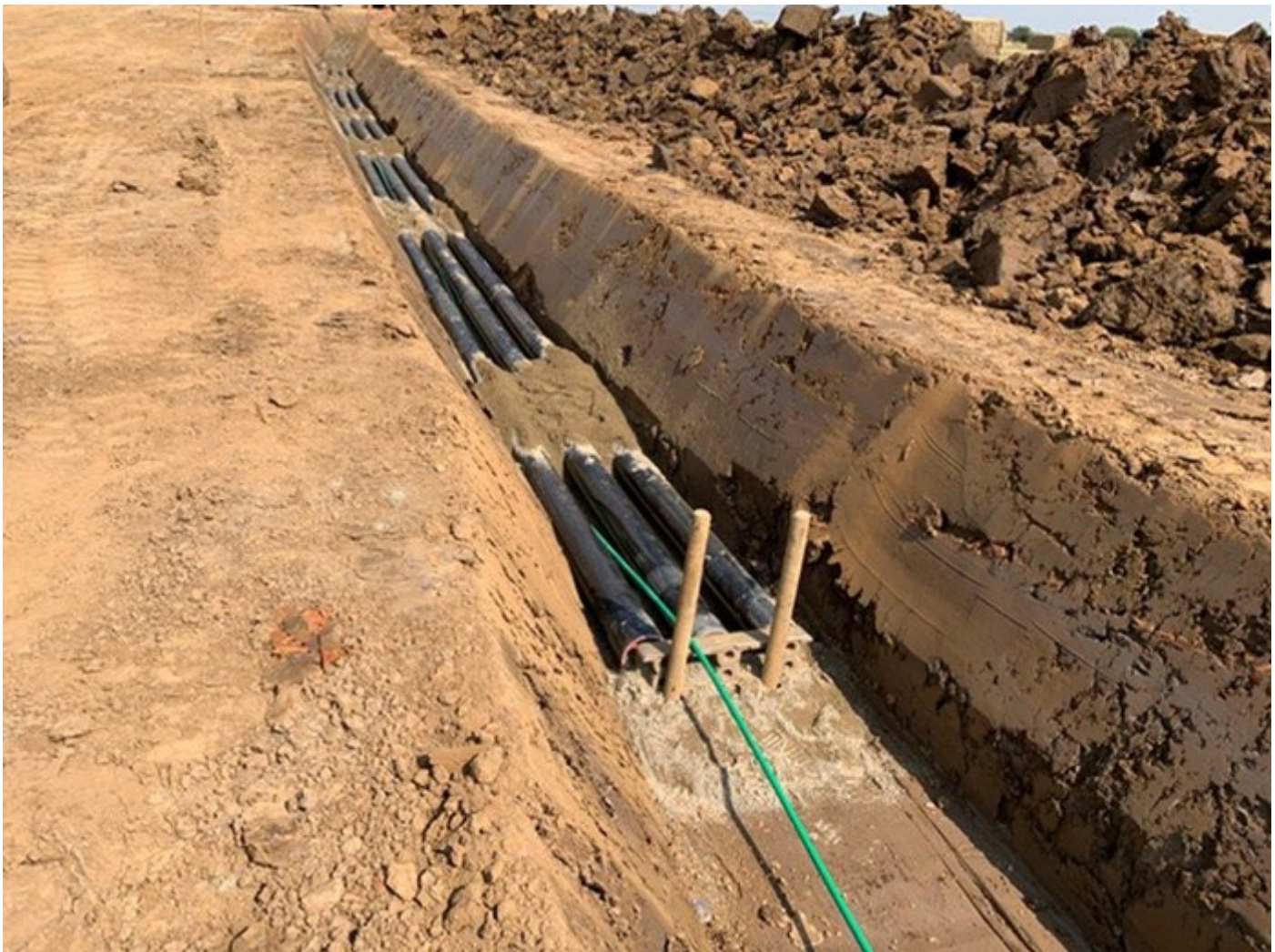
Figure 3.18: Example of an onshore export cable trench.
