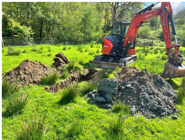
Figure A1 - Excavation of test pit TP1
