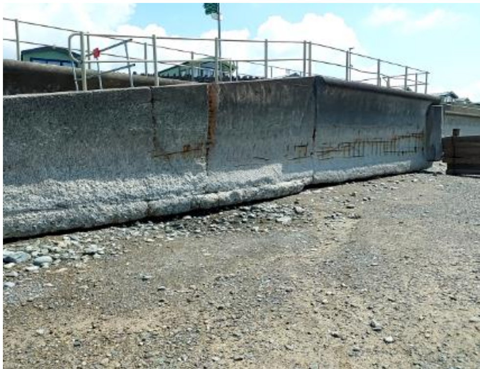
Figure 2: Slipway retaining wall erosion damage.
