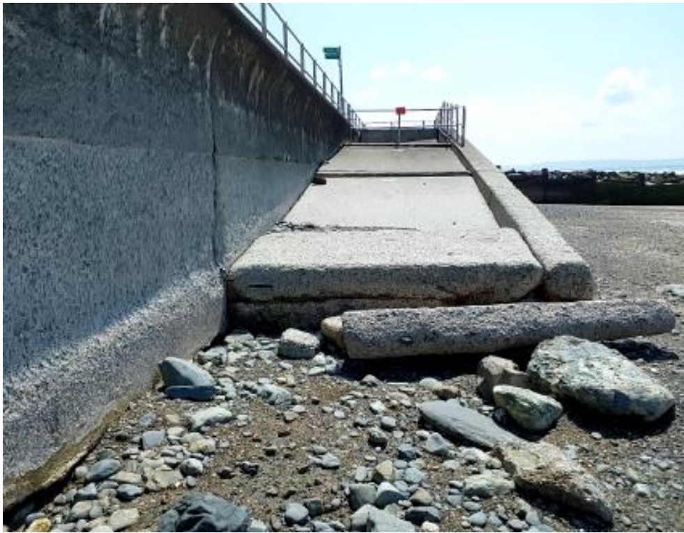
Figure 1: Tywyn Neptune Road slipway damage
