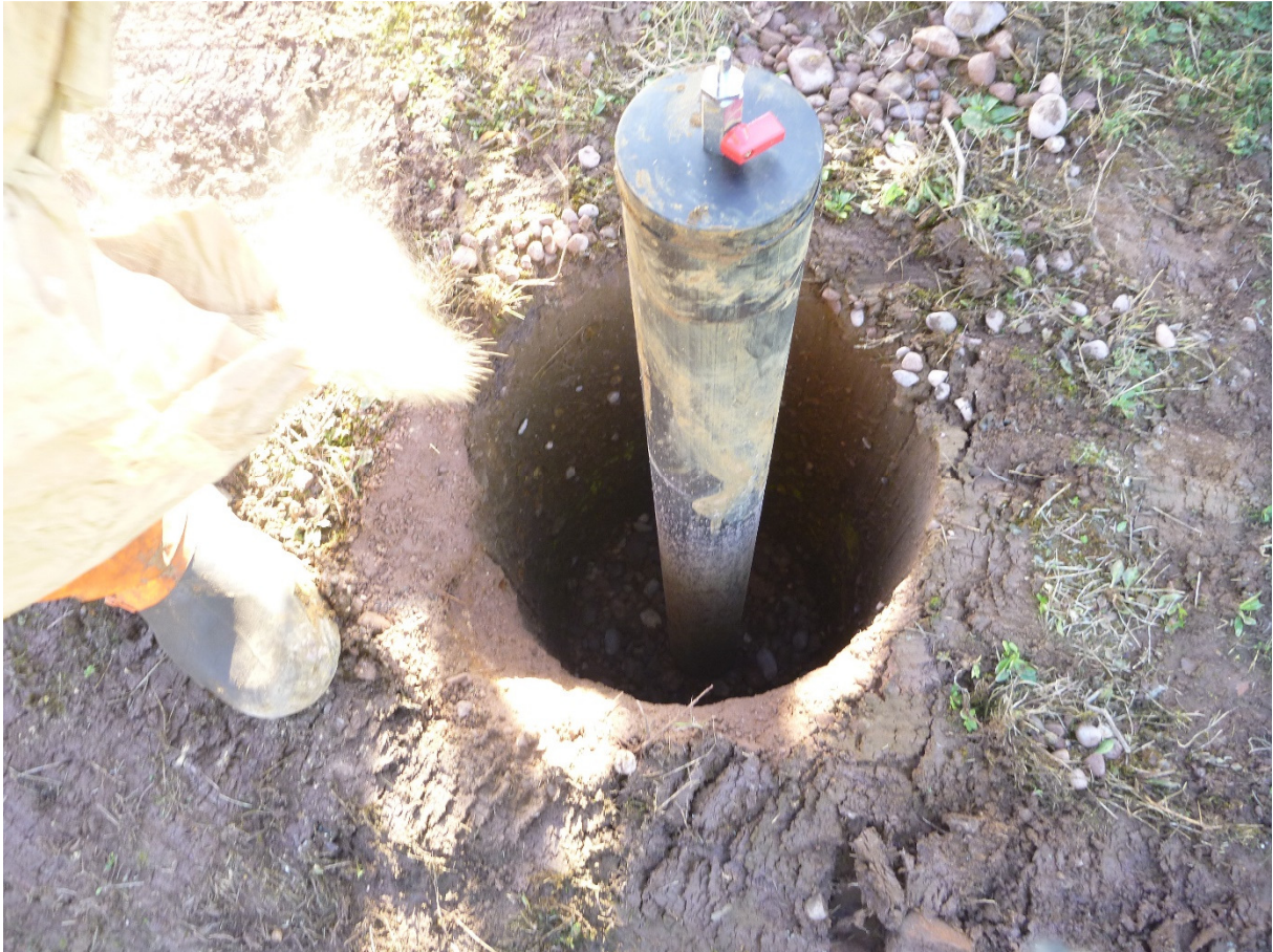
Photograph 3: Sealing the gravel back with dry bentonite prior to filling the annulus with hydrate bentonite slurry
