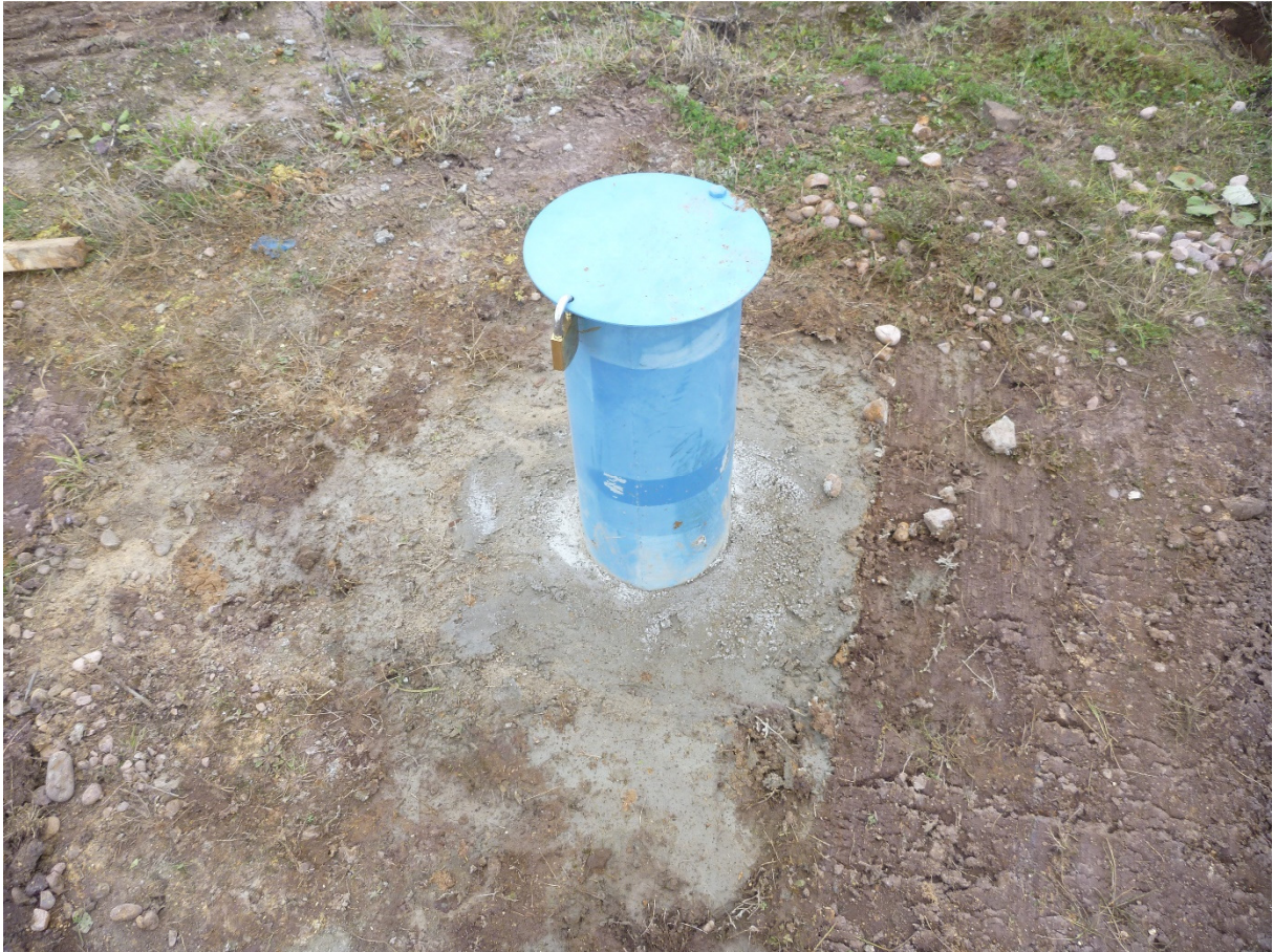
Photograph 4: Completed borehole, with concreted, lockable steel cover
