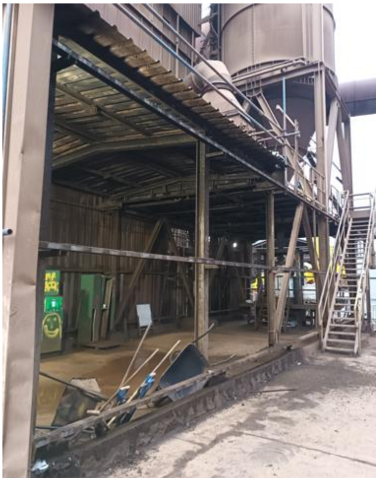
Photograph 4-2: Existing building under refurbishment (with cladding removed)
