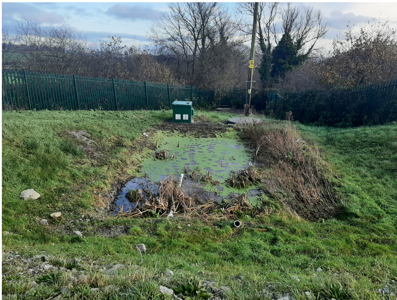
Above: Reed bed with pump housing to rear.
