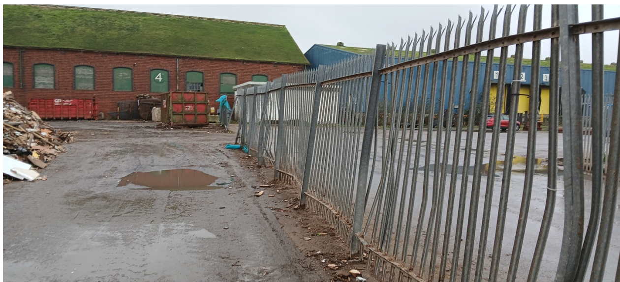
Photo 7 - Perimeter fencing at SWWP Ltd, Newport
