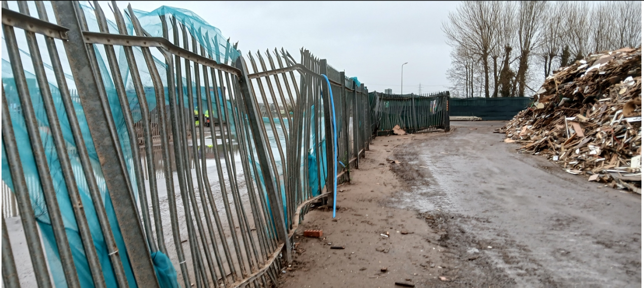
Photo 8 - Perimeter fencing at SWWP Ltd, Newport
