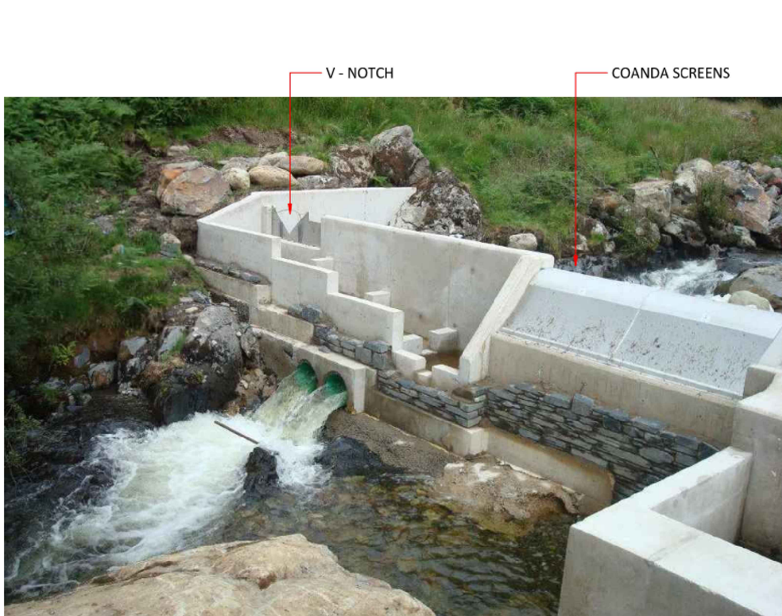
WEIR: Micro Hydro, 375kW Cadair Hydro (150m head, 300l/s, pelton turbine), operated by Dragon Hydro www.dragonhydro.com Photos: Jonathan Bensted
