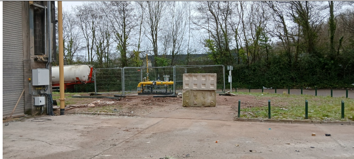
Photo 4 – Showing the new gas pipe that has been installed ready to heat the dryer
